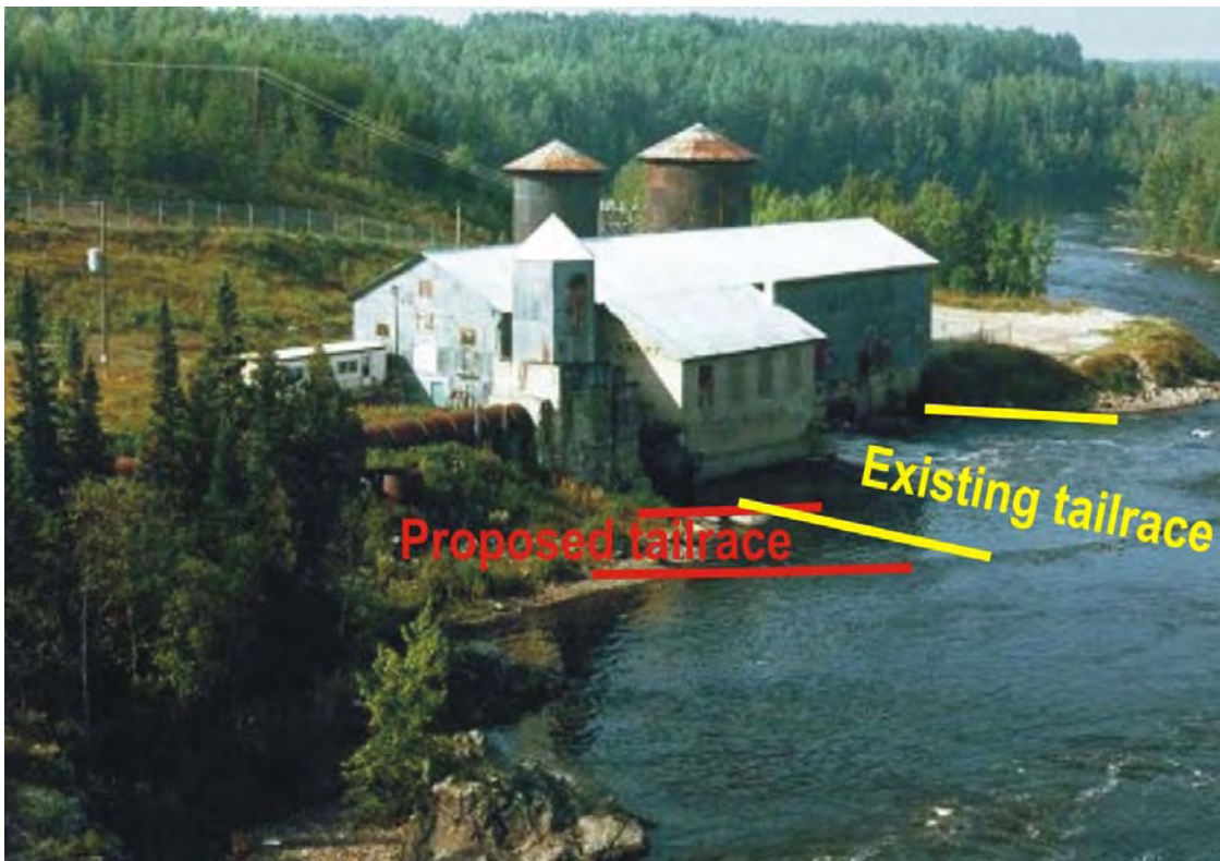
Photograph 4-6: Sandy Falls GS Existing Tailrace and Approximate Location of Proposed Tailrace
