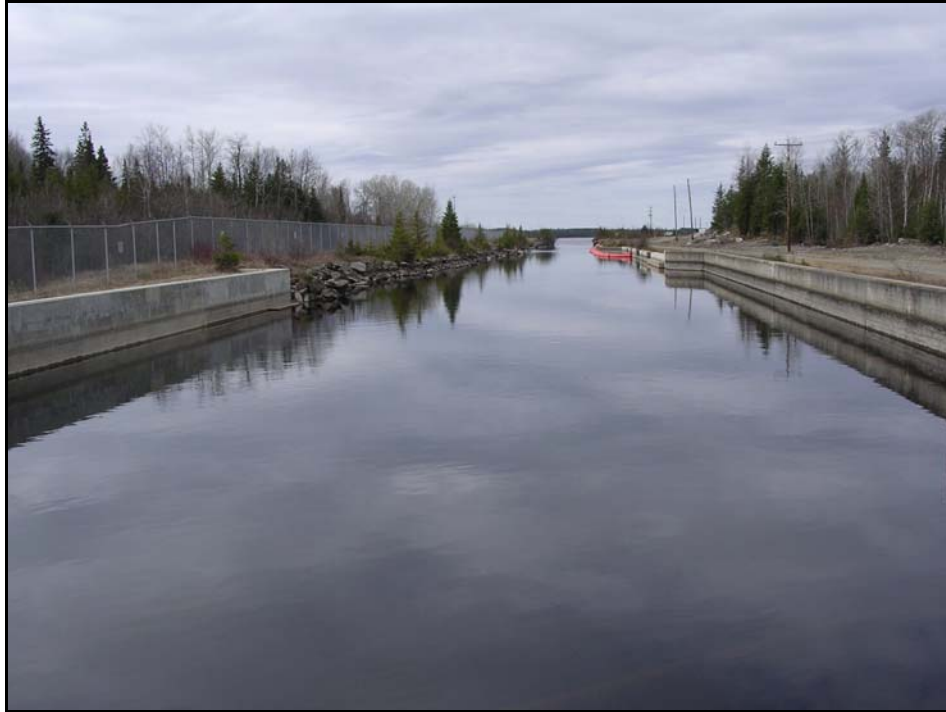
Photograph 1: View of intake channel looking upstream from the top of the penstock, April 22, 2005. Area in foreground will be temporarily isolated with a cofferdam and de-watered.
