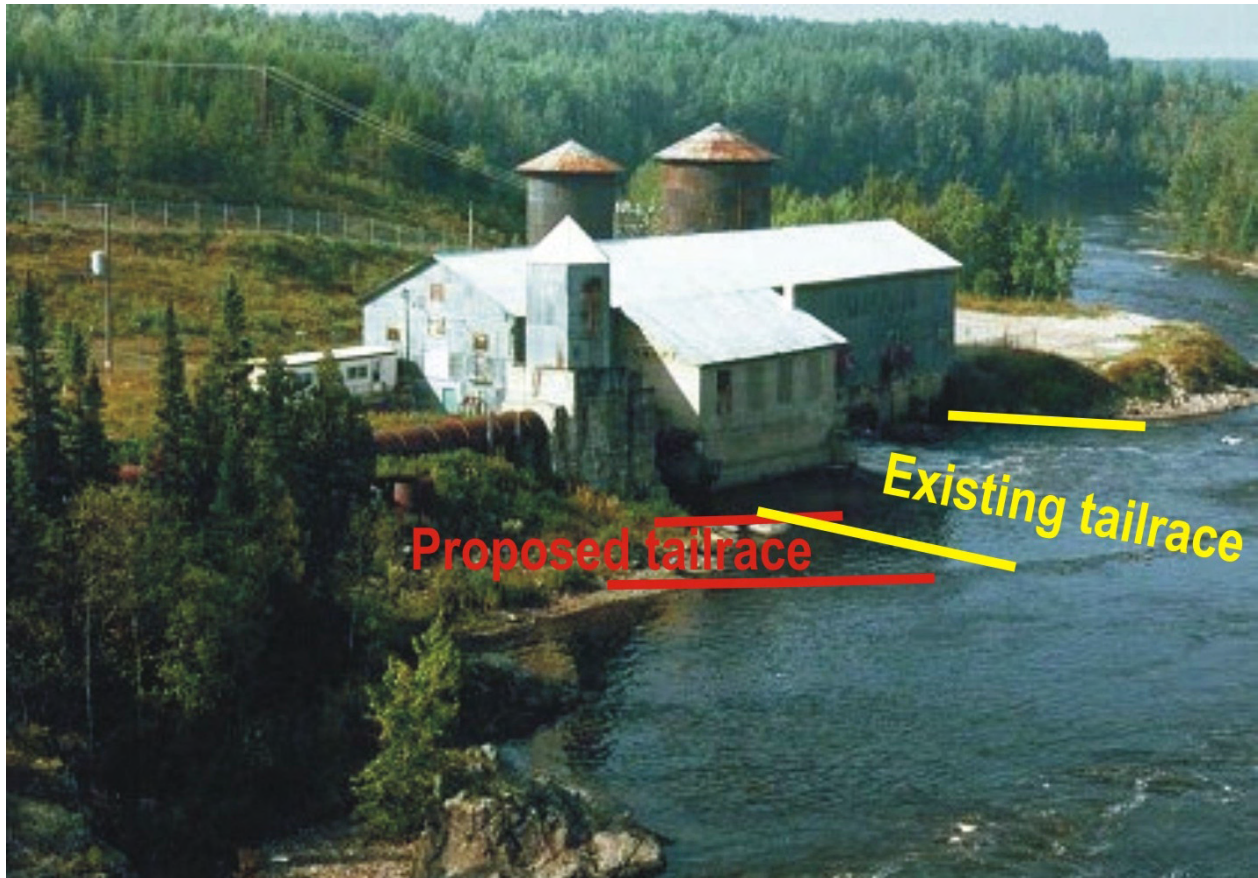
Photograph 1.6: Sandy Falls GS Existing Tailrace and Approximate Location of Proposed Tailrace
