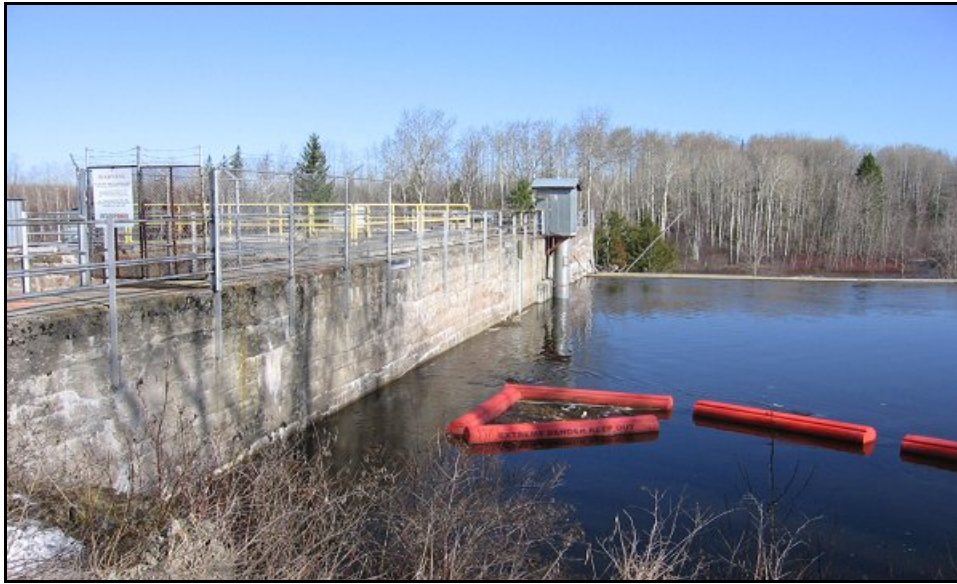
Photograph 1: View of intake structure and area to be temporarily isolated with a cofferdam and de-watered.
