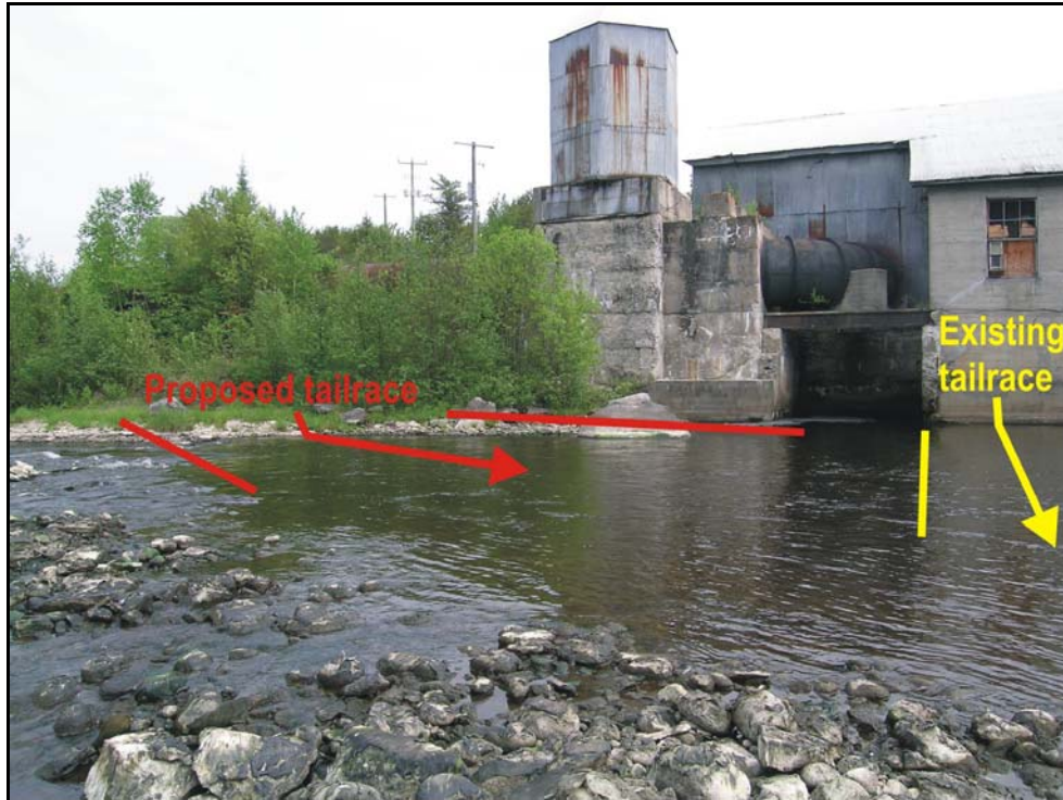
Photograph 3: View of the proposed tailrace location at Sandy Falls GS, from the existing cobble shoal that has developed along the upstream edge of the existing tailrace. June 8, 2005.
