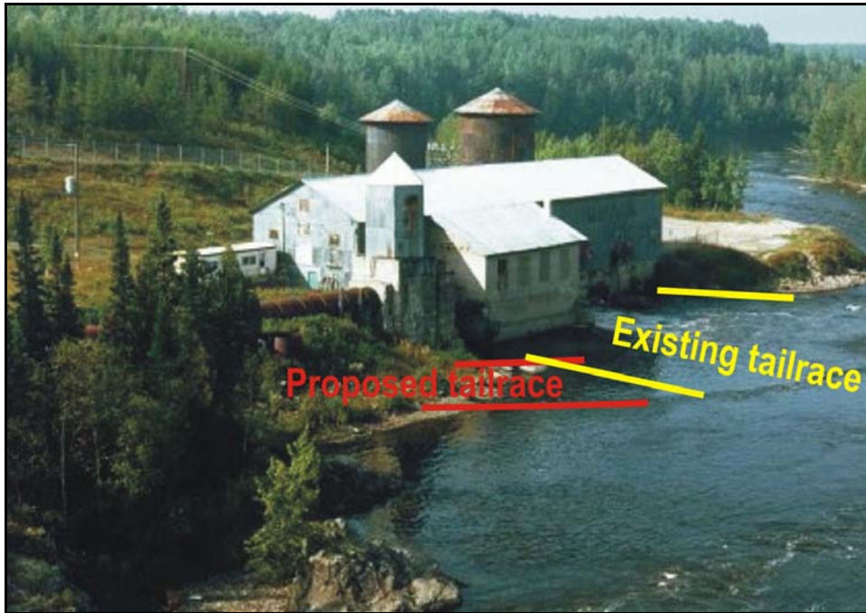
Photograph 2: Downstream view of Sandy Falls GS showing the existing tailrace and the approximate location of the proposed tailrace.
