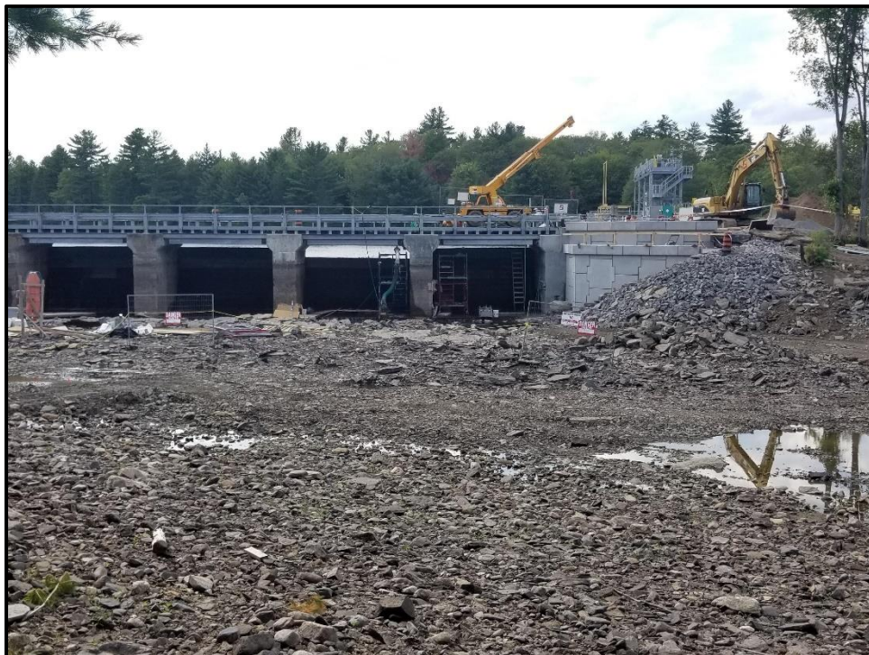
Photograph 28. Forebay De-watered for Maintenance, Looking Towards Bridge (2018-08-24).
