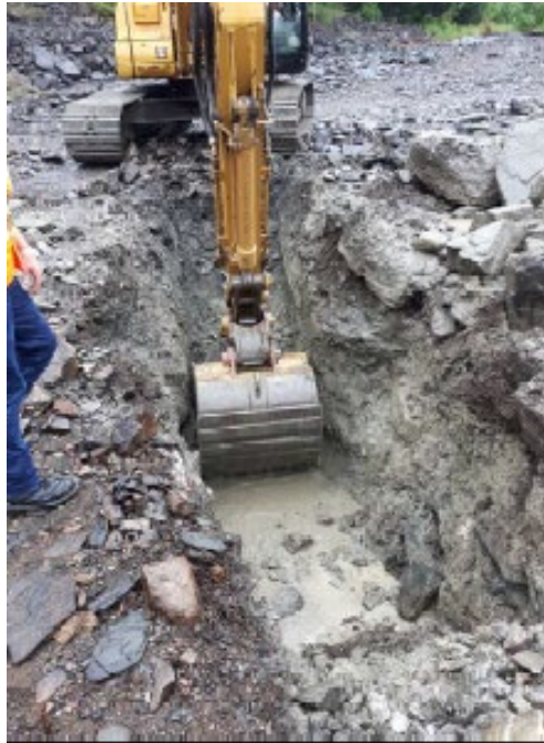
Figure 3-4. Excavator at One of the Test Pits in the Forebay
