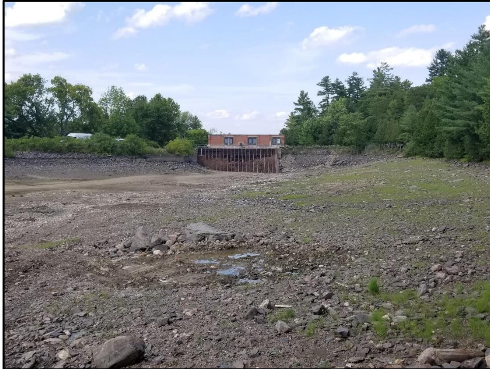
Photograph 27. Forebay De-watered for Maintenance, Looking Towards Trash Racks and Generating Station (2018-08-24).
