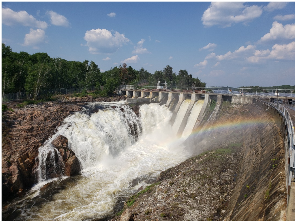
Figure 3-4. Looking upstream at the spillway and sluiceways at the Stinson GS on July 2, 2019 under higher flow conditions than present during field investigations in 2020 (OPG supplied photo, see Figure 3-2 for approximate location).
