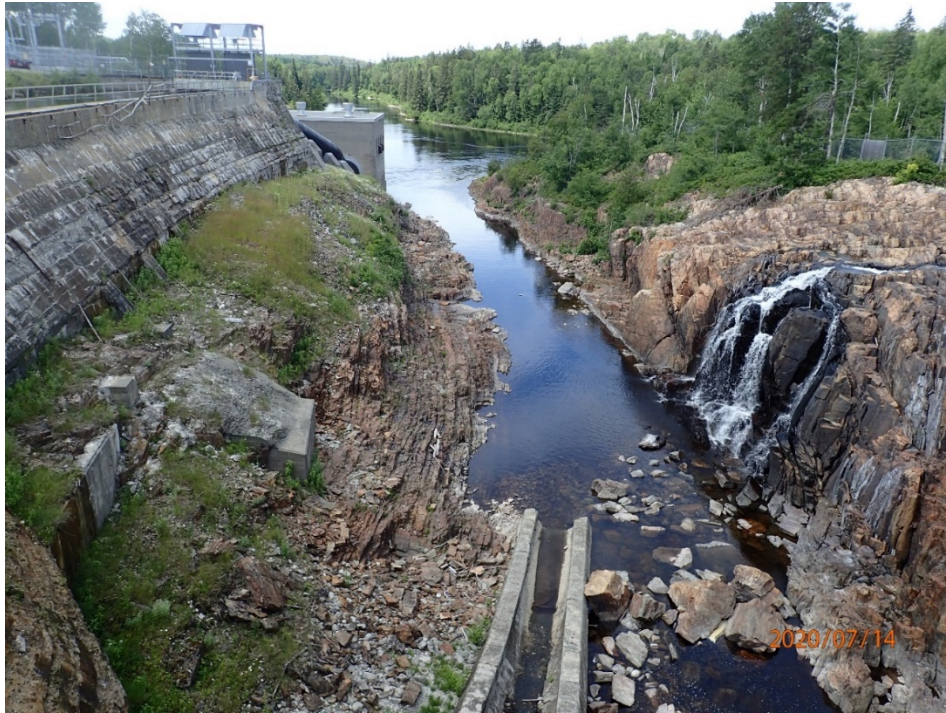
Figure 3-4. Looking upstream at the spillway and sluiceways at the Stinson GS on July 2, 2019 under higher flow conditions than present during field investigations in 2020 (OPG supplied photo, see Figure 3-2 for approximate location).
