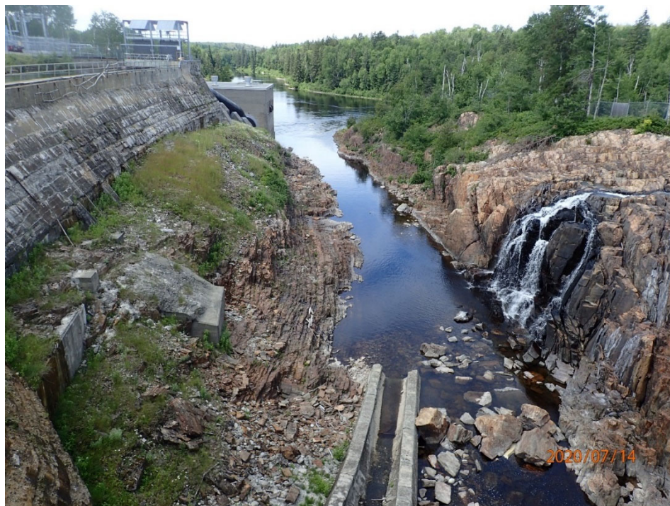
Figure 2-6 Stinson Spillway: Leakage Flow Only
