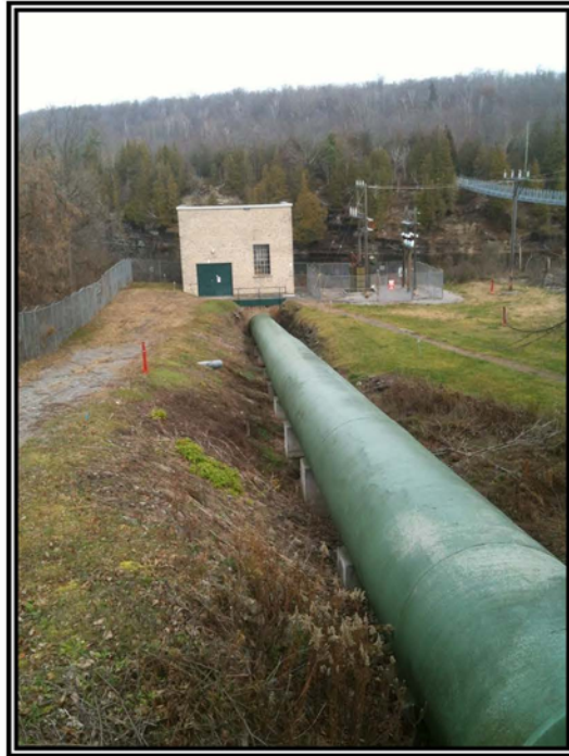
Image 6: View to Northeast of Lower Site (Trent River in Background), including Secondary ("Pup") Powerhouse, Access Ramp, Small Transformer Yard, and Penstock.
