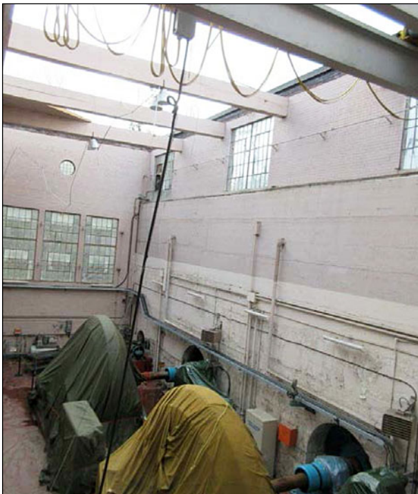
Figure 28. The loss of the roof exposed the interior of powerhouse and equipment to the elements, notably heavy precipitation associated with the storm [KGS Group, 2018].
