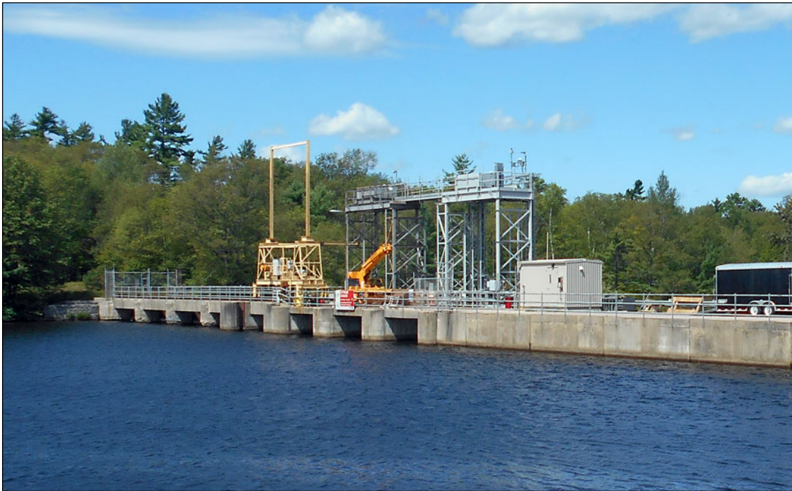
Figure 18. The main control dam is located on the South Branch of the Madawaska River. Originally containing five, stoplog sluices, an additional three gate sluices were added in 1968.
