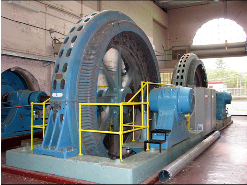
Figure 23. The Calabogie GS contains generating units connected to quadruple-Francis horizontal turbines.
