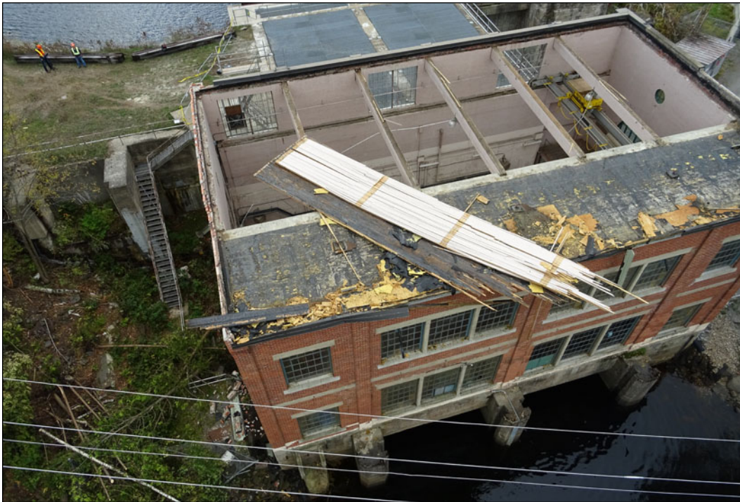
Figure 26. The storm on September 21, 2018 dislodges a significant portion of the powerhouse roof [OPG, 2018].
