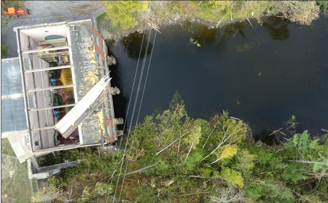
Figure 15. The 2018 tornado damaged not only the powerhouse but also numerous trees in proximity to the building [Arcadis, 2018].
