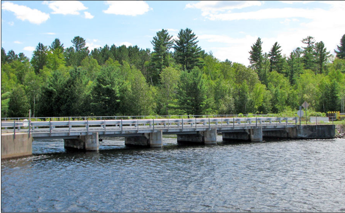
Figure 19. An entrance dam, also known as a cutoff dam, with five sluiceway controls the flow of water into the forebay.
