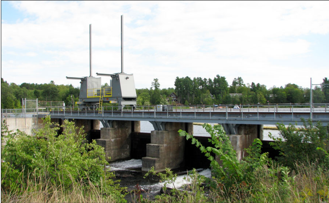
Figure 17. A concrete dam with five, stoplog sluices controls the flow of water into the North Branch of the Madawaska River.
