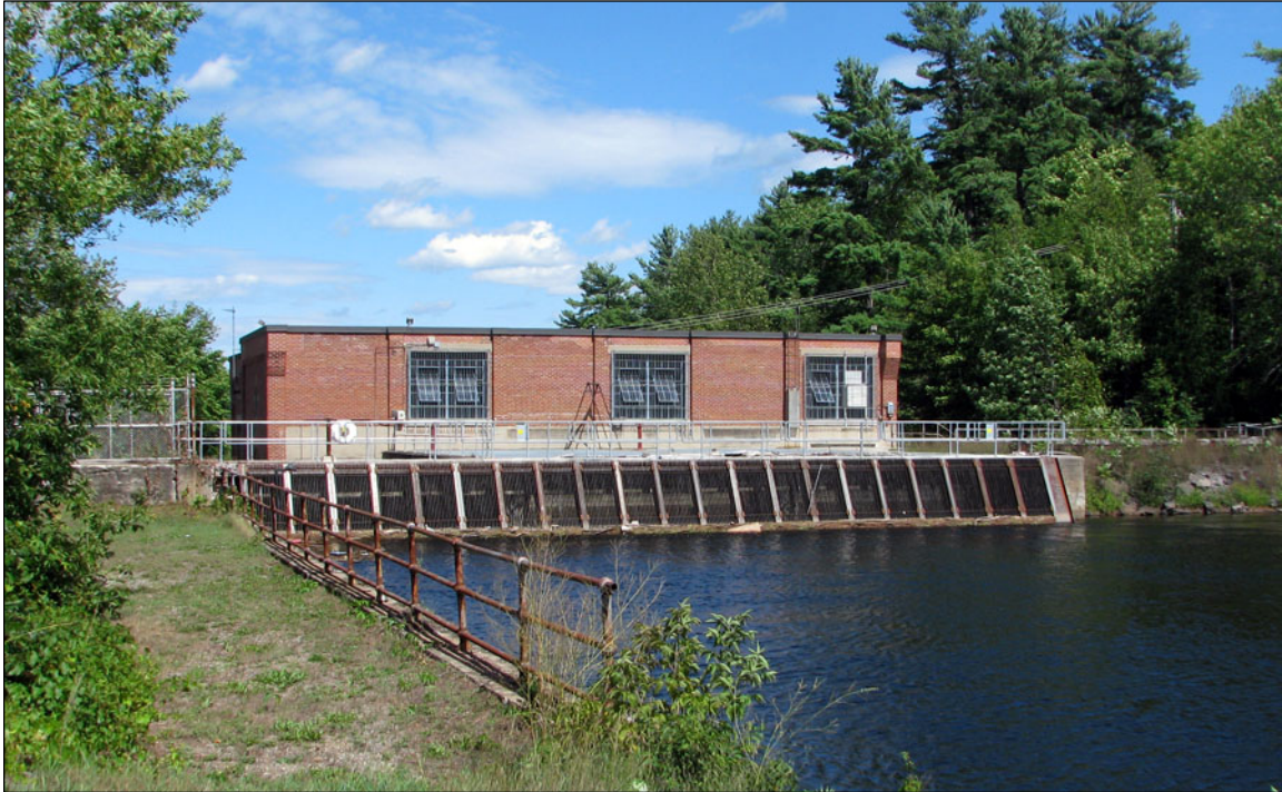
Figure 21. Trash racks extend across the upstream face of the headworks that house the turbine wheel pits.
